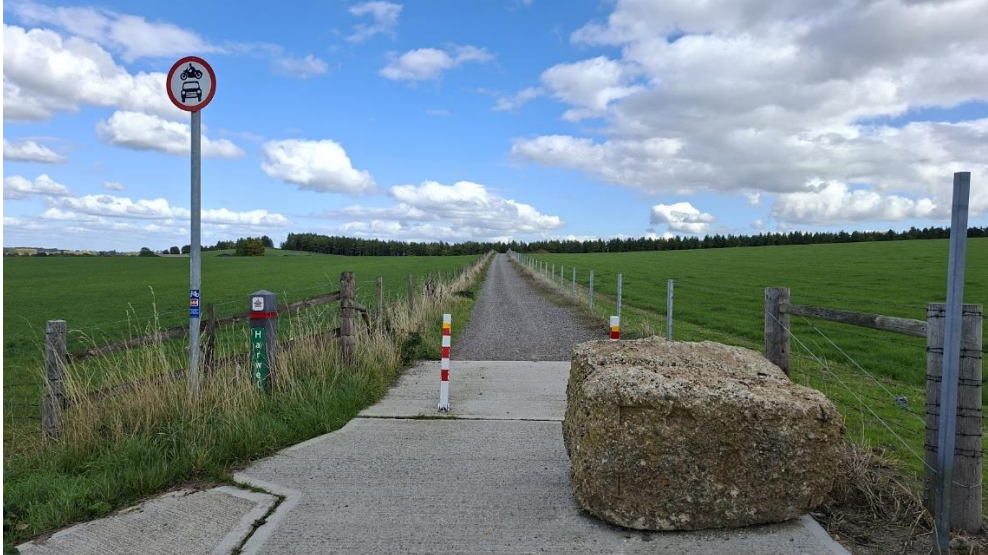
Icknield Greenway near Ginge - bollards width of only 59.5 inches (1.51m) and a boulder obstructing the approach (under TRO?)
