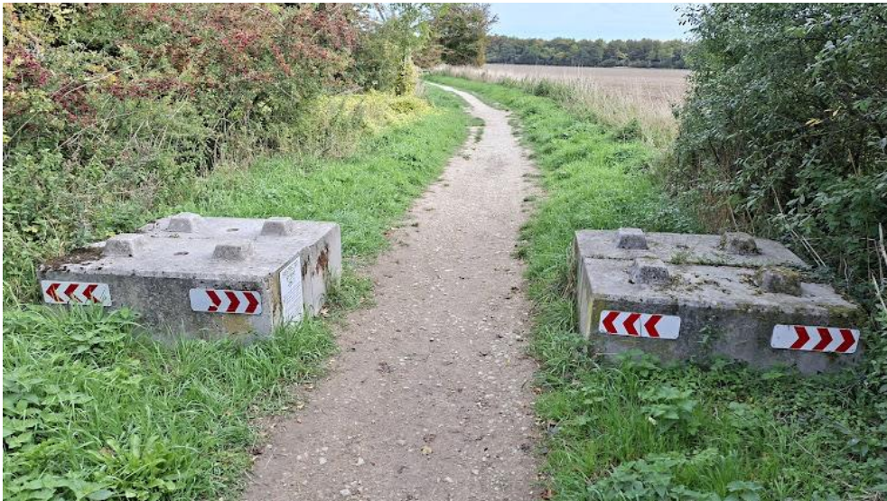
OCC Section 66 obstruction on the Ridgeway National Trail near Ashbury - gap width of only 61.5 inches (1.57m) - under TRO?
